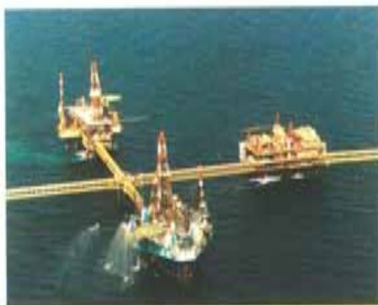
Qatargas Offshore Facilities
